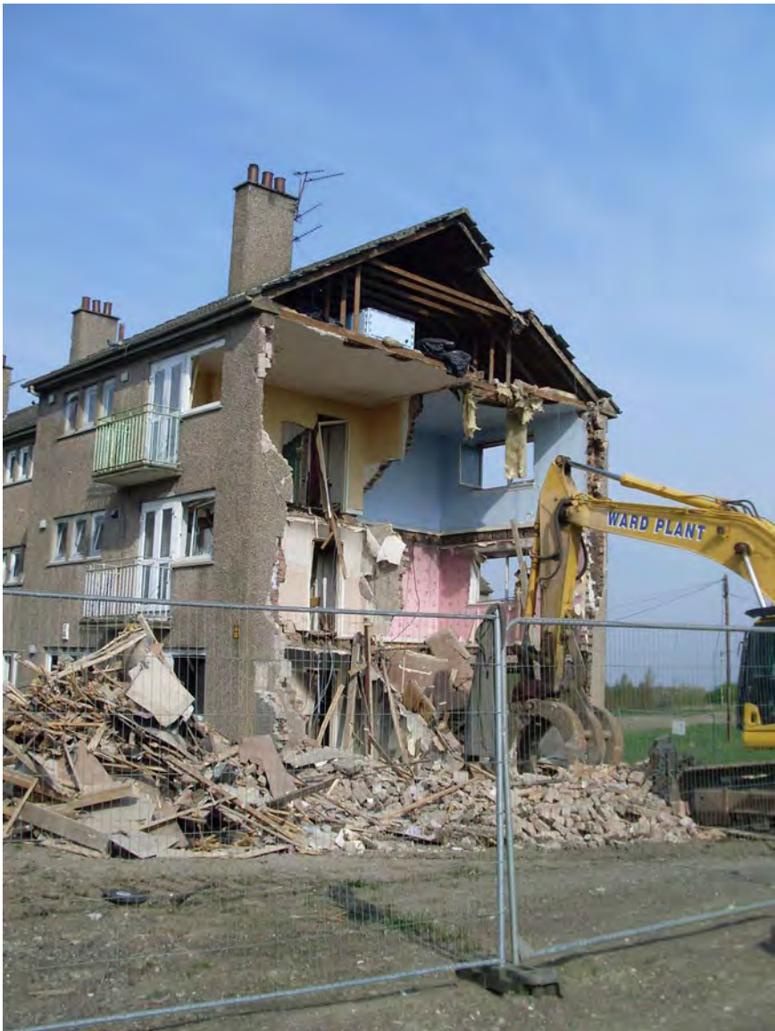
Figure 7.1 Demolition in Easterhouse, 2009.
