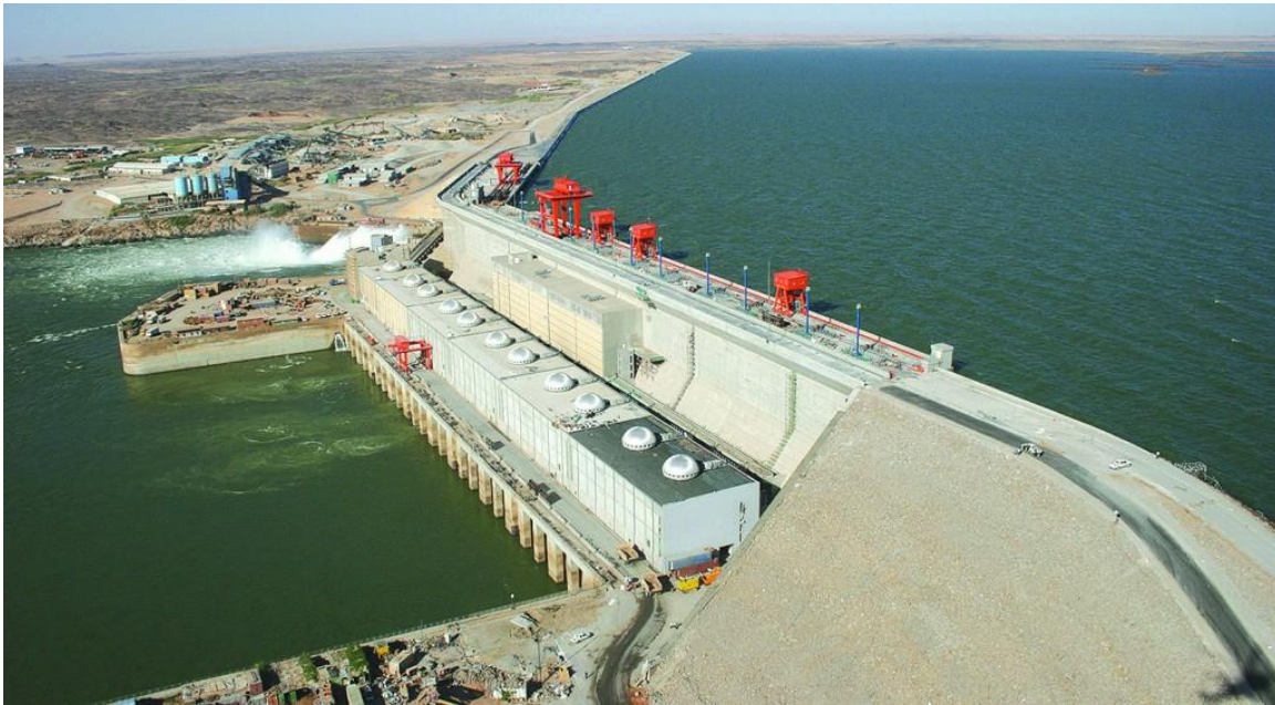
Figure 2.2. The Merowe Dam and its reservoir.
