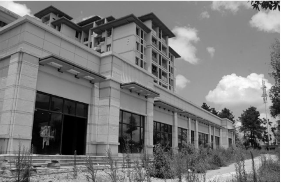
Figure 7.4. Decaying relocation housing in Gui'an New Area. (Photograph by Tim Oakes.)
