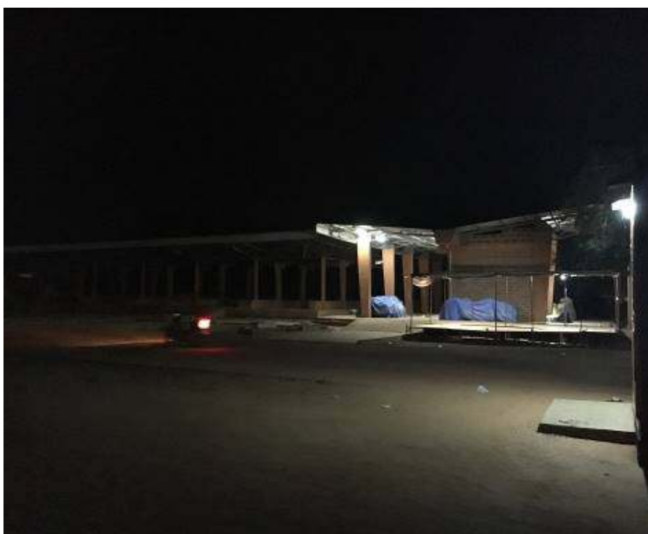
67 Service eau potable
